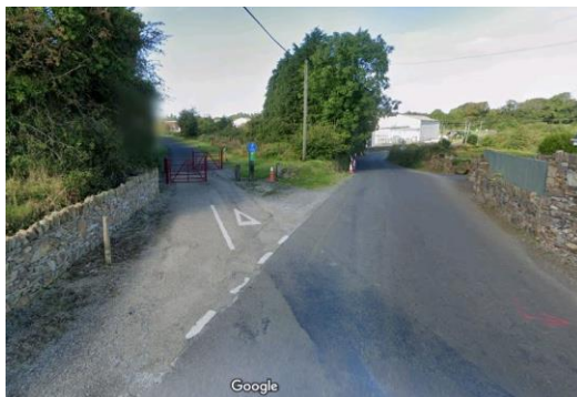
Figure 46 The Waterford Greenway crossing a public road
