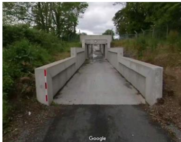
Figure 47 The Waterford Greenway going under a private lane
