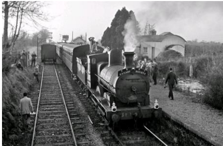
Figure 3 Palace East Station (Joanes, 1963)
