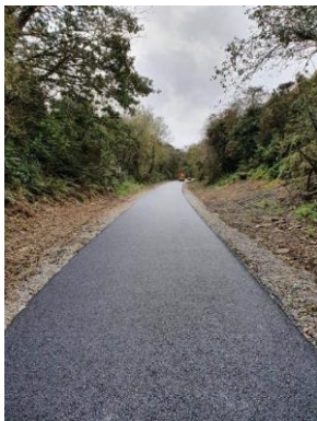
Figure 5 South East Greenway under construction (Harney, 2021)
