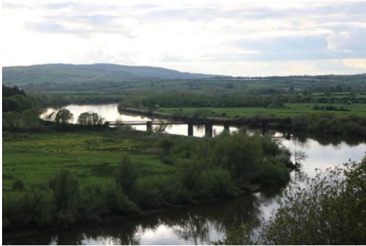
Figure 10 The Railway Bridge over the River Barrow at New Ross
