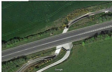
Figure 48 The Waterford Greenway going under a dual carriageway
