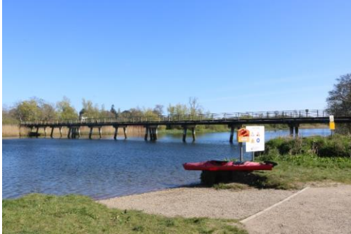
Figure 27 Edermine Bridge over the River Slaney
