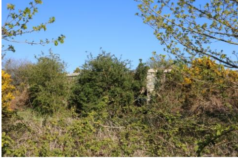
Figure 21 The overgrown Ballybrennan's Bridge
