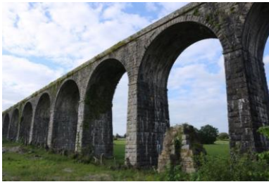
Figure 55 The Borris Viaduct, part of the proposed Barrow Valley Greenway
