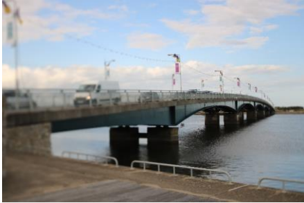
Figure 33 Wexford Bridge over the River Slaney
