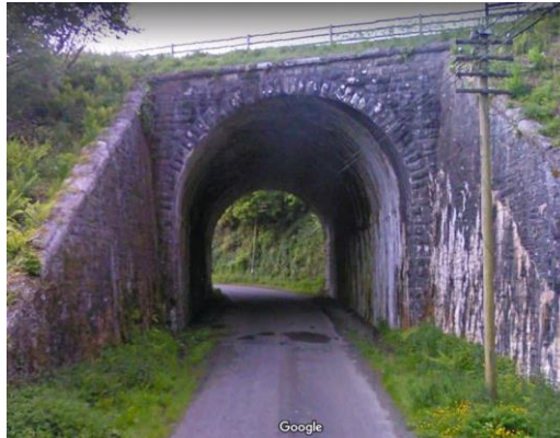
Figure 12 One of the arches under Ballyanne Bank (Google Street View)
