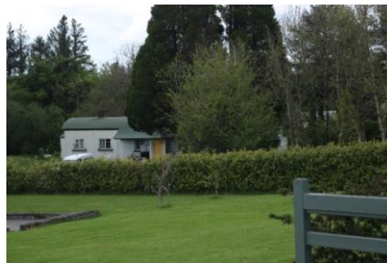
Figure 15 Palace East Station
